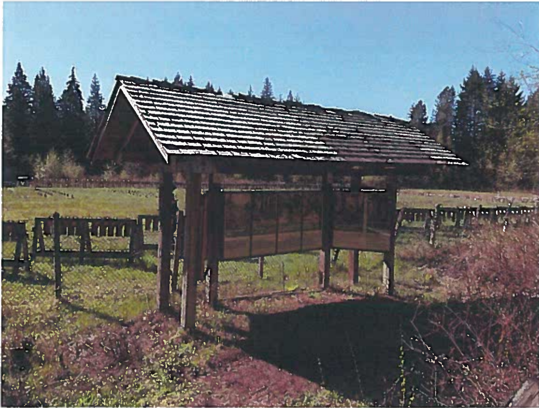
Figure 6. The sign shelter after 15 years of exposure in Maple Ridge.
