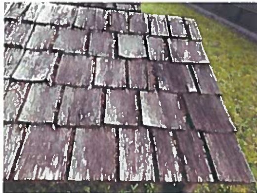
Figure 4. Untreated western redcedar shakes after 24 years of exposure in Vancouver.
